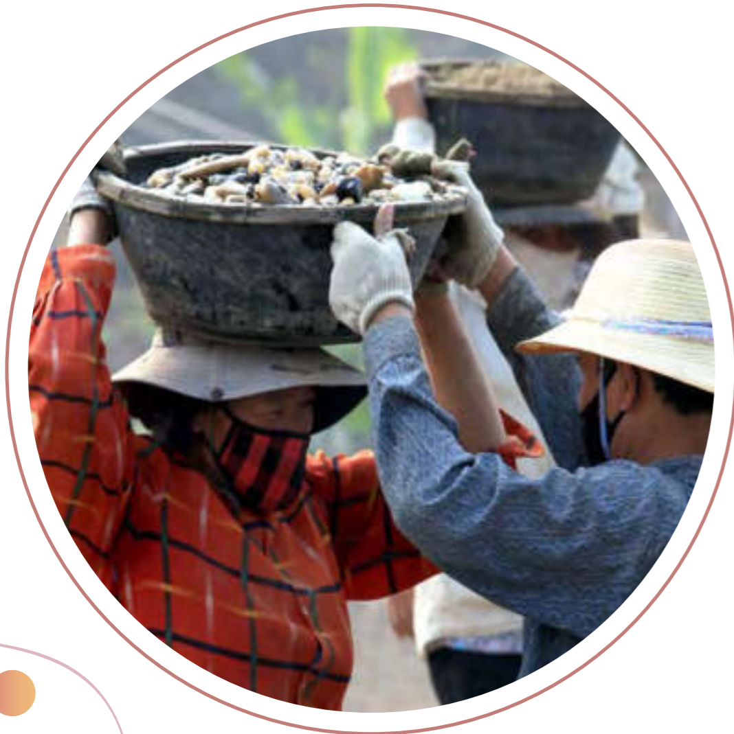
Construction workers at work. Source: ILO/Truong Van Vi
