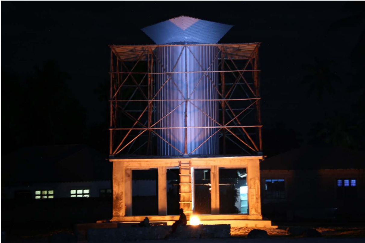
Figure 5: Wind water tower in Michamvi, Zanzibar
